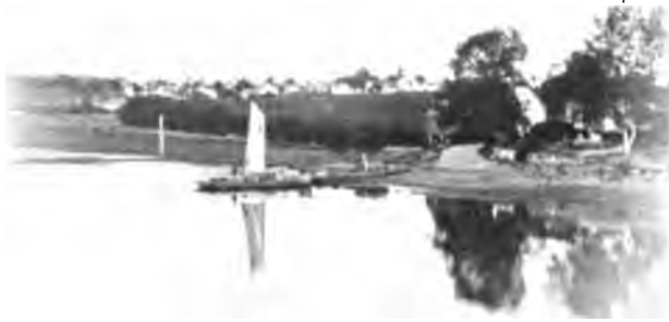
THE FERRY LANDING, RICHMOND SIDE.
